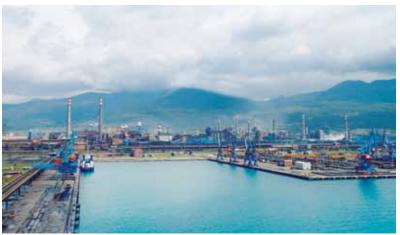
Production process commences, as the raw material is brought to the plants. Coal is shipped to the coke plants to be subjected to the coking process whereas fine ore is shipped to the sinter plant for the sintering process.
